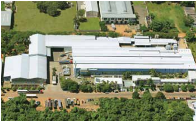
Above: Brazil Bauru Plant
